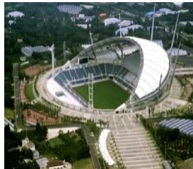
[Unique roof and cladding]
